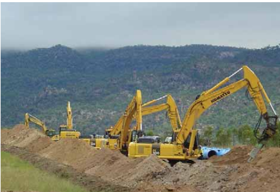
Burdekin-Moranbah Pipeline construction
