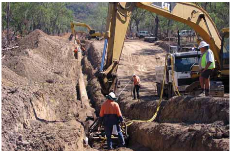
Construction of the Stag Creek Pipeline
